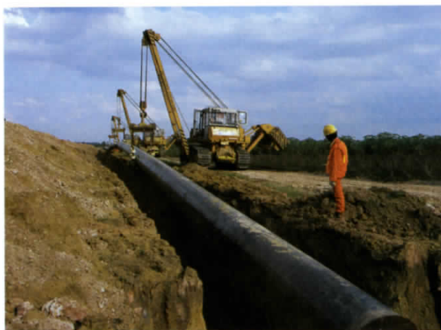
Figure 2. Pipeline lowering.
