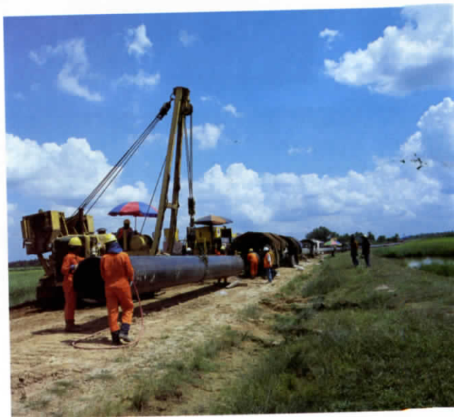
Figure 4. Pipeline welding in progress.
