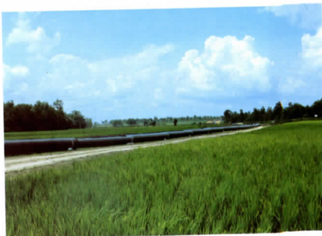
Figure 5. Pipe string along ROW through paddy fields.
