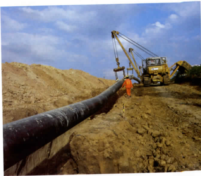
Figure 3. Pipeline lowering at elevation.
