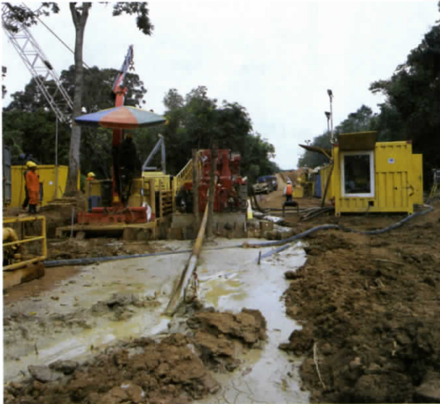
Figure 1. Horizontal directional drilling at site.
